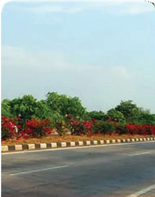
Highways/ Municipal Road
